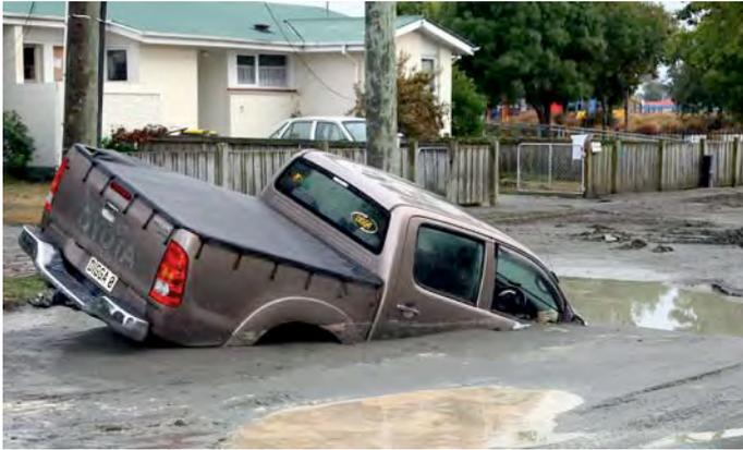
Roads in Christchurch, New Zealand's second city, suffered liquefaction damage.
