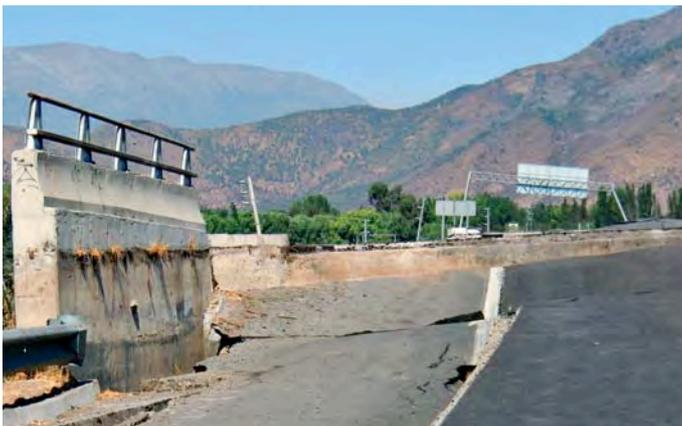
Lateral spreading and subsidence made many roads impassable, like this bridge outside Talca, 255 km south of Santiago.
