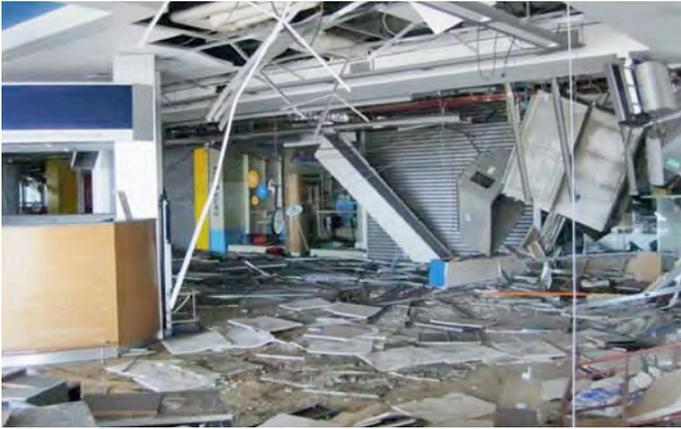
The main building itself at Santiago International Airport withstood the quake safely, although non-structural elements were badly damaged.
