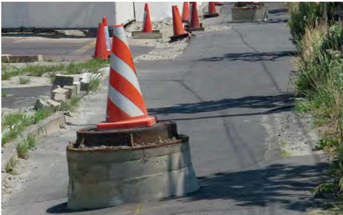
Protruding manholes are a typical sign of subsidence damage in reclaimed land areas (here: Tokyo Bay).
